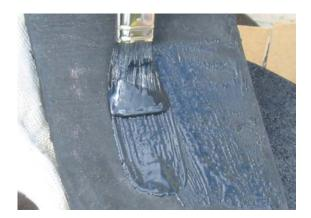
5) Apply a second coat to both surfaces and allow to dry until slightly tacky (approx. 10 minutes @ 25°C). In the event of over-drying, apply a third coat.
